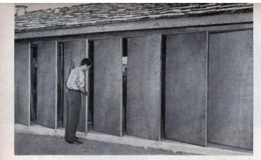
Bedroom wall consists of slab doors permanently set at a stagger. Movable glass panes will be between
