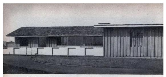
"House of the 21st Centruy" has rustic shake roof and board-and-bat siding. Makeshift fence is only temporary
